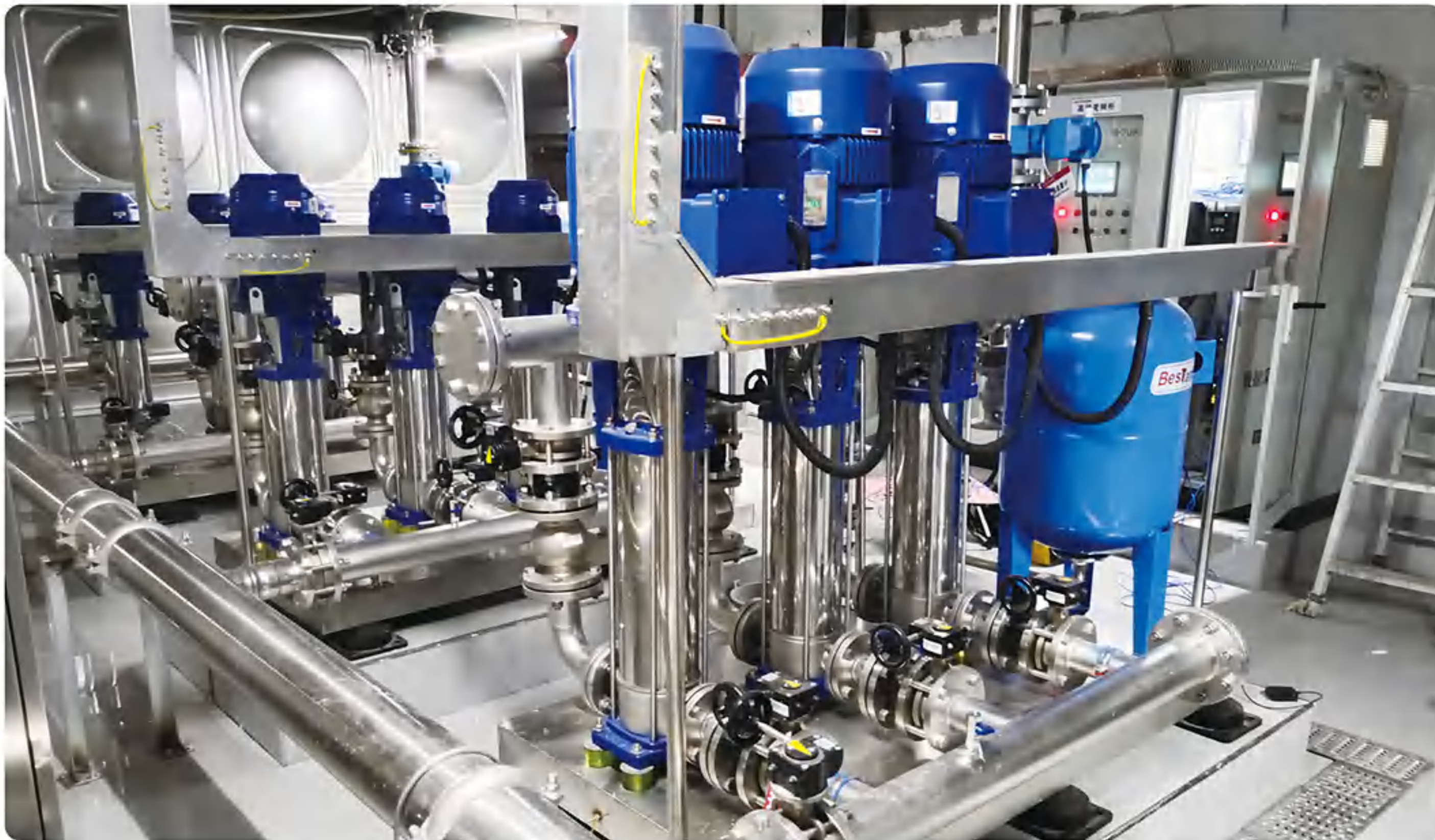
Ximeng Longrun Construction Engineering Co., Ltd. Project Engineering
