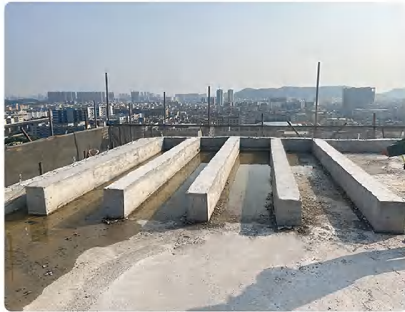
1. Make cement foundation
