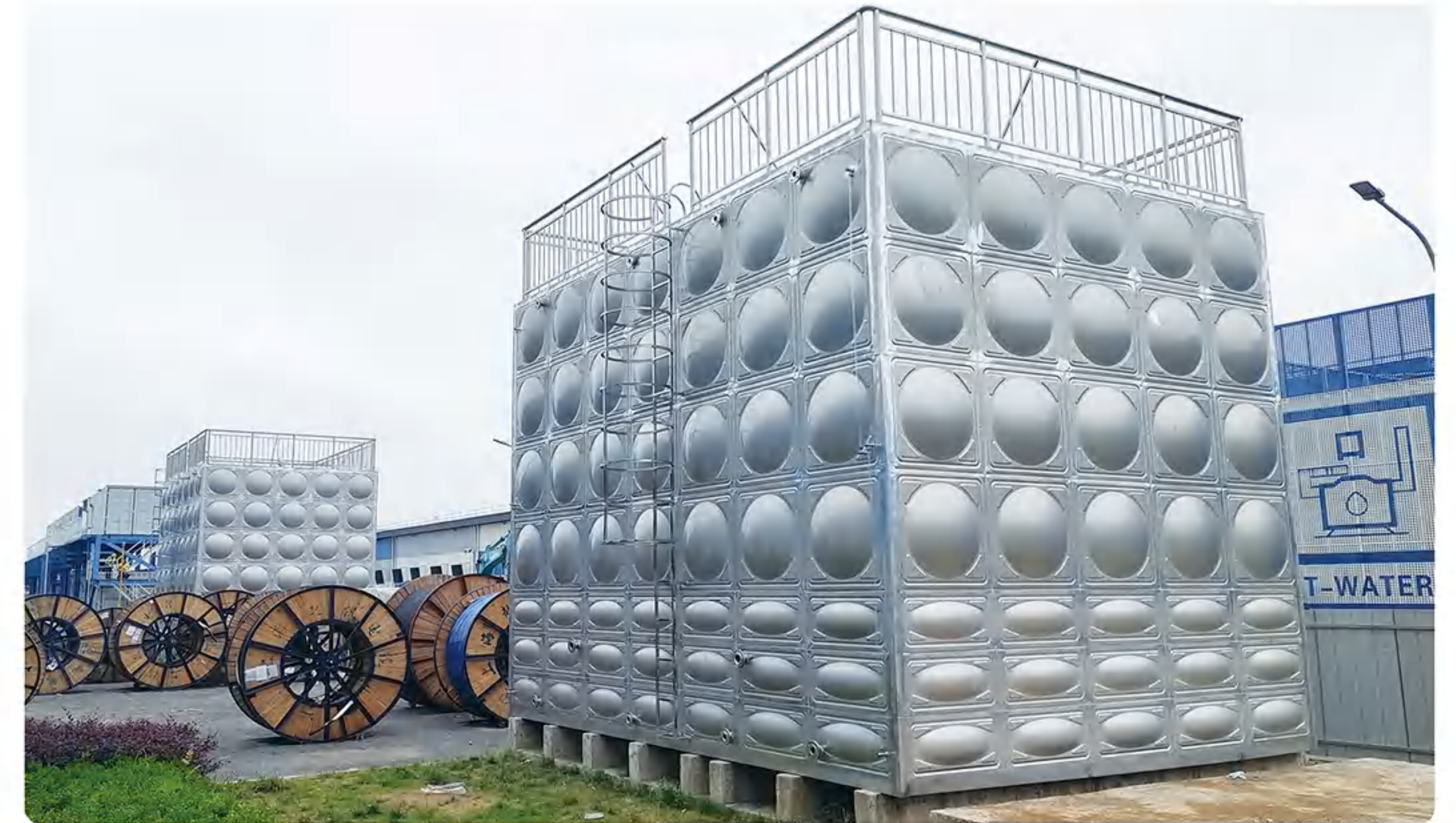
FUJIAN TONGTIAN CONSTRUCTION ENGINEERING CO., LTD. 600 TONS WATER TANK
