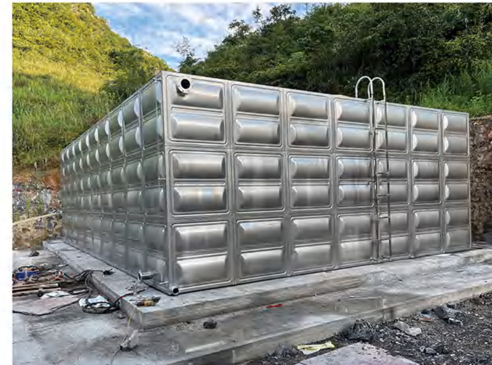
210 ton water tank in Chengmai County, Hainan Province
