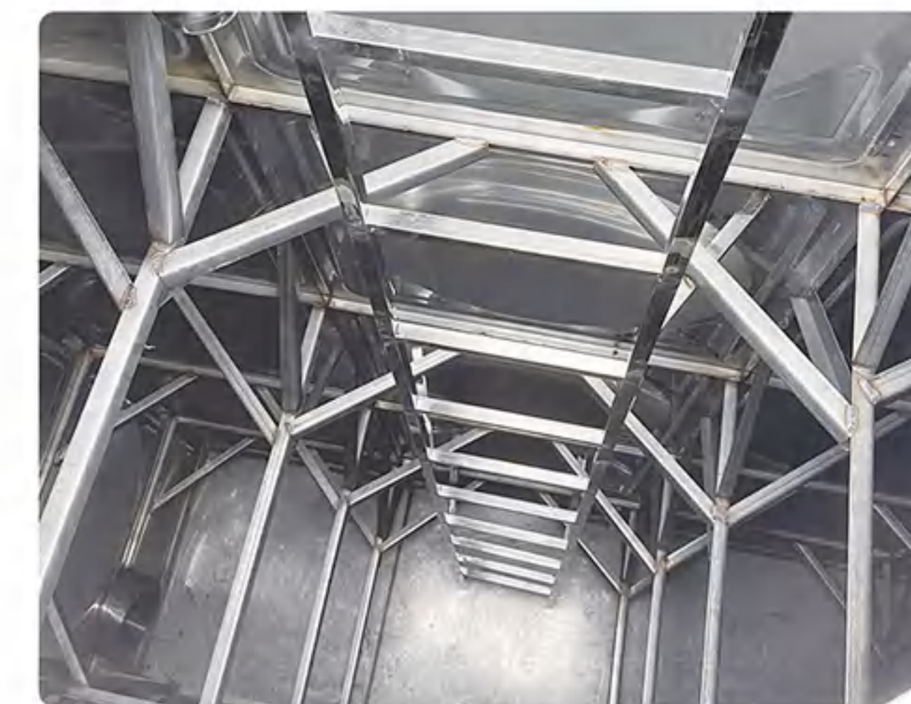
11. Install internal and external ladders
