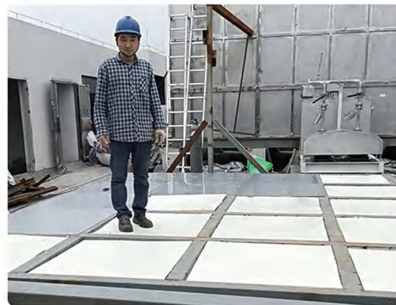
4. Laying the upper base plate
