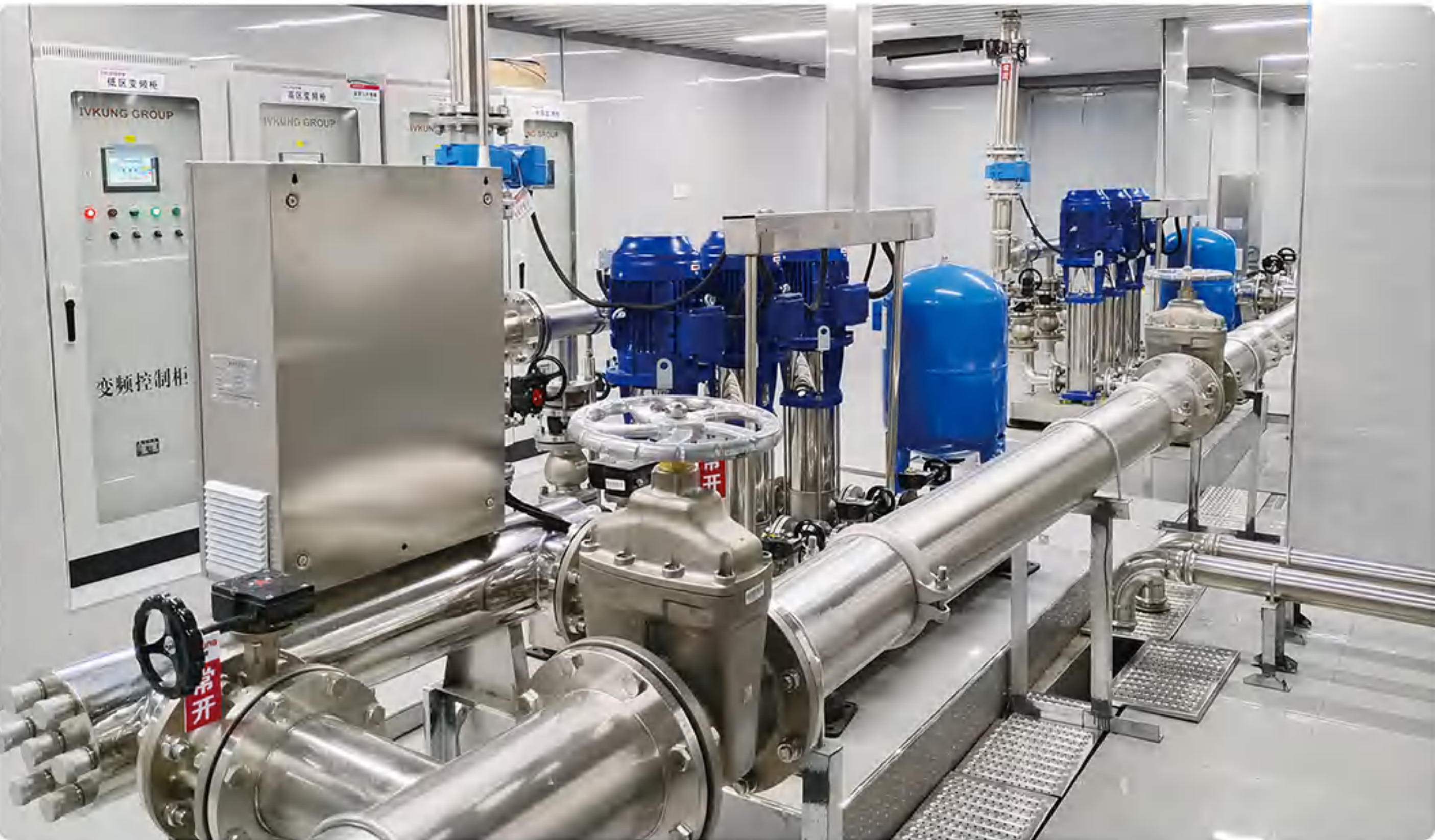
Shanyang County Zhongyu Dingli Mining Co., Ltd. Project Engineering
