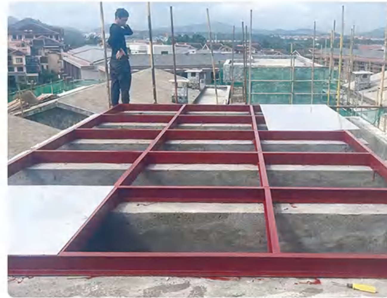
2. Welding Channel Steel
