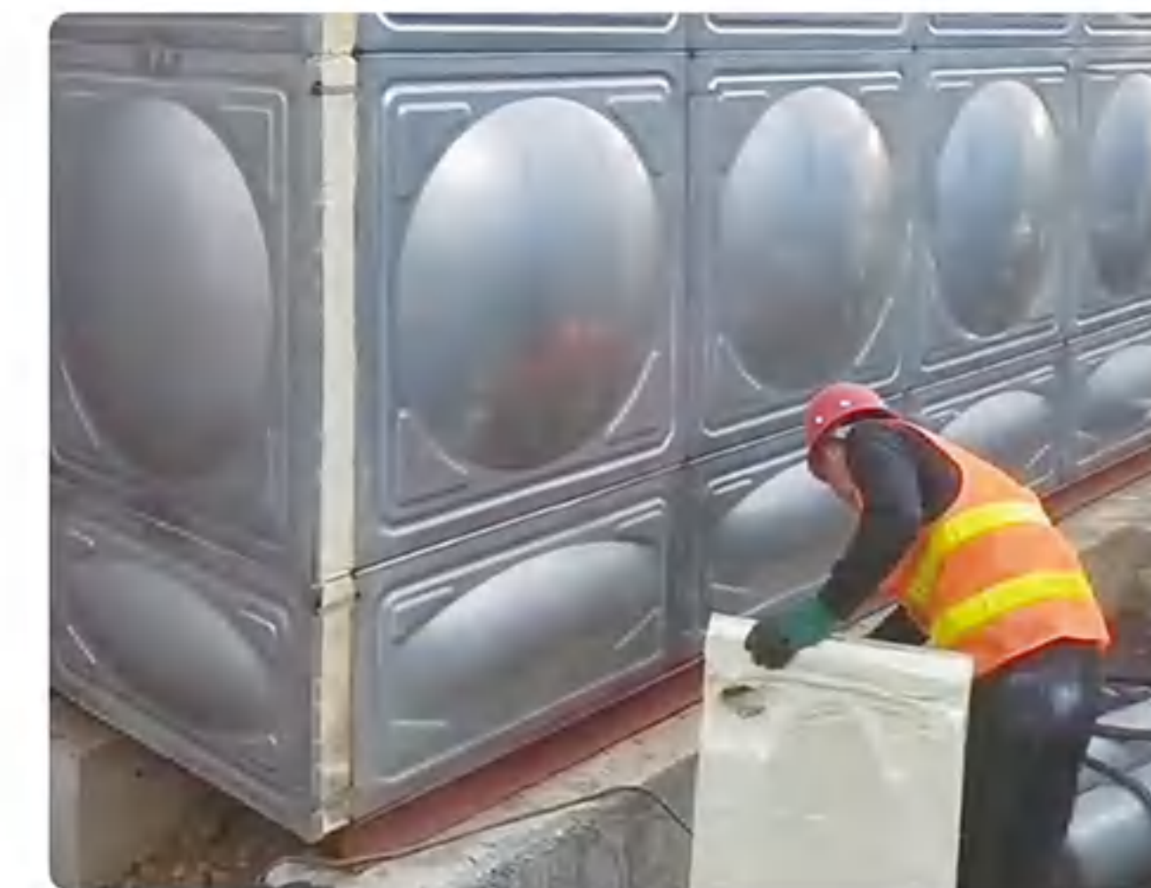
9. Welding insulation outer panels
