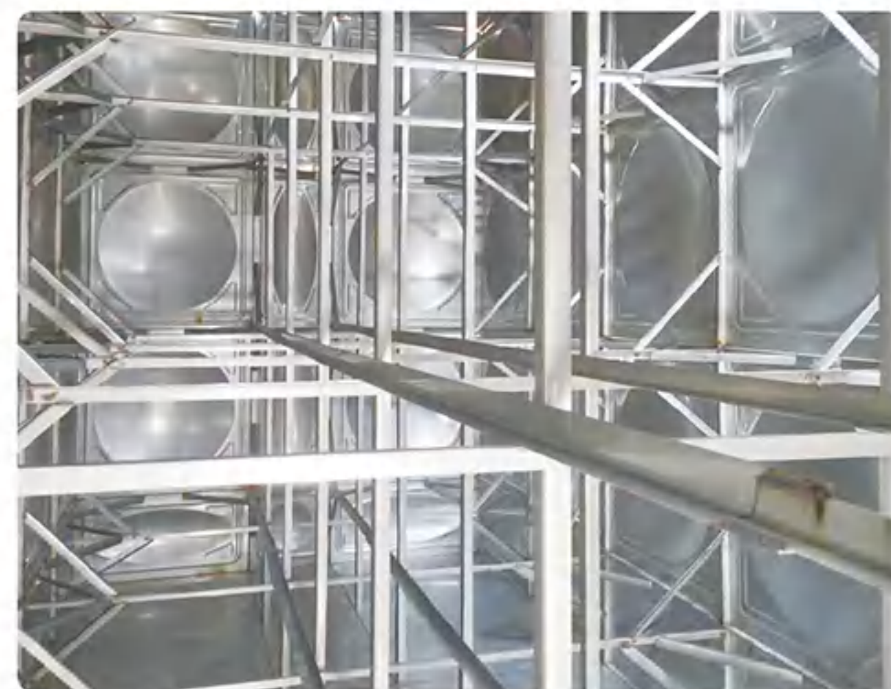
6. Install horizontal and vertical reinforcement
