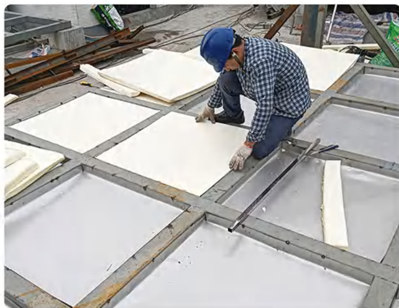
3. Install the bottom plate and lay the insulation layer
