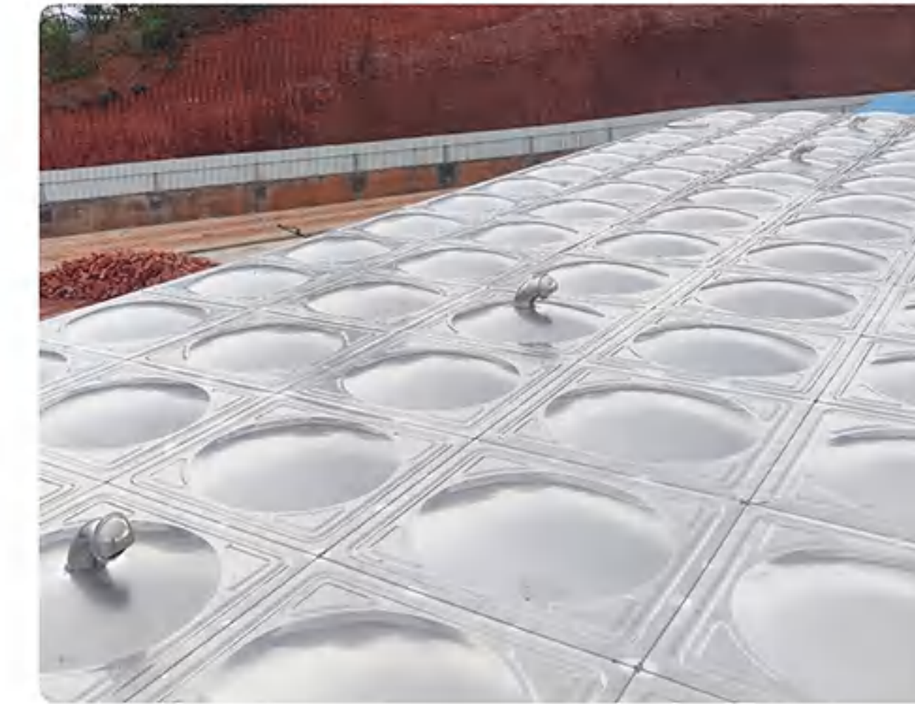
7. Install the top plate
