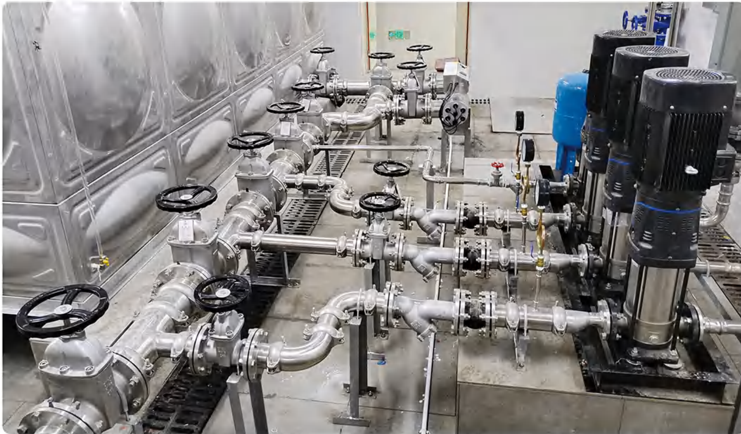
Wuzhou Ruyou Printing and Dyeing Co., Ltd. Project
