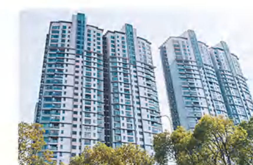
High-rise building pressurized water supply
